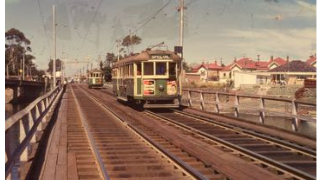
Footscray Tram 670 on Tram only bridge over Maribynong River FB
