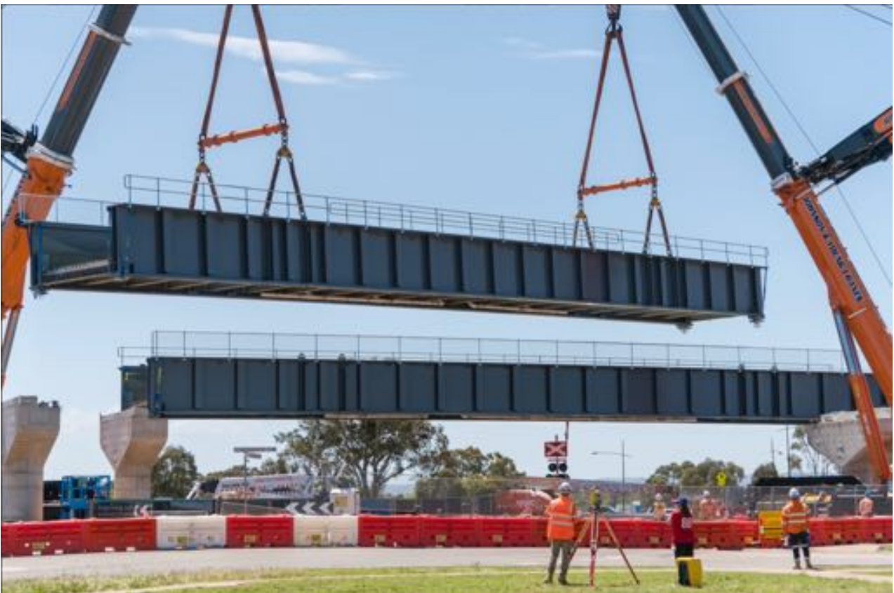
The second steel bridge being lifted into place at Coburns Road, made of steel because of long span diagonally across road, concrete would be too heavy presumably. Bigbuild website 2025 | I
