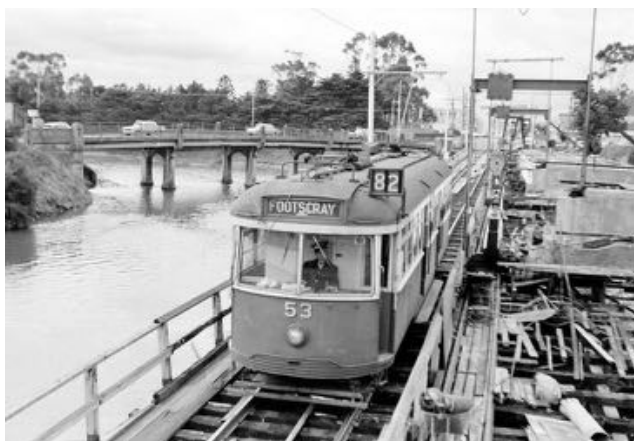
Footscray Tram 53 crossing Maribynong River Tram Only bridge one track being rebuilt Road Bridge in Background FB 20210905
