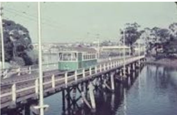
Footscray Tram on Maribynong River tram only bridge FB 20210905
