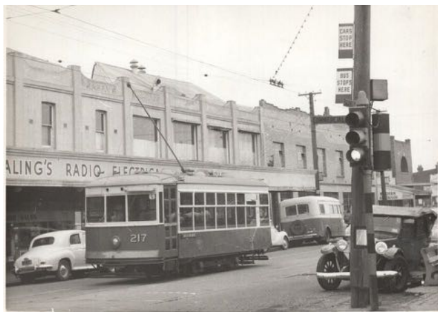
Barkly St, Commercial Rd beside Primary School 217 FB 20210905
