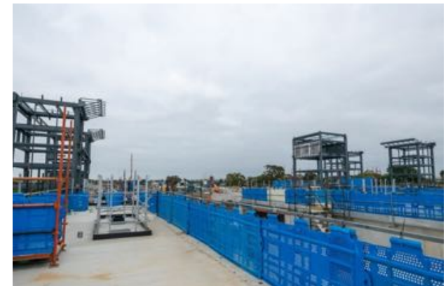
Lift shafts at Melton Bigbuild website 202511
