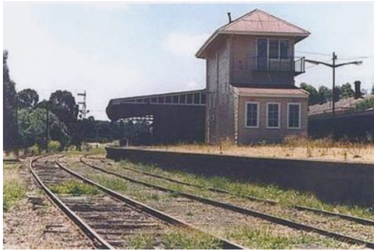
Castlemaine Station Platform 3, Yard & Castlemaine A Box prior to the start of track restoration March 2001 VGRSG
