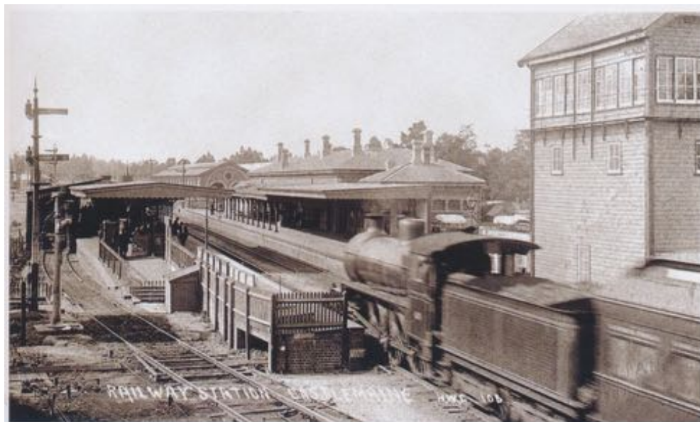
Castlemaine Station 1912 Bendigo Bound possibly the Great Northern Limited, loco is a new A2 4-6-0 express passenger loco in Canadian Red Livery with white lining. VGRSG
