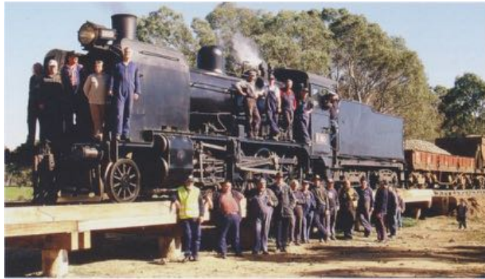
First train K160, over newly rebuilt Walmer Road Bridge 27-06-2002
