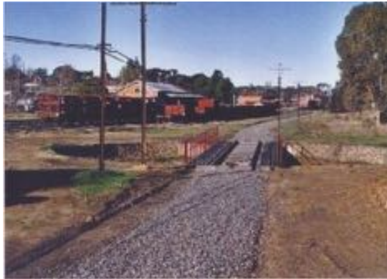
Base prepared for new Turntable that was moved from Woodend VGRSG
